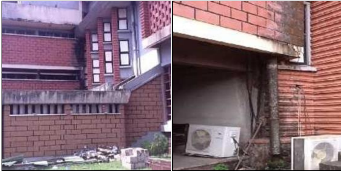
Figure 9 Deterioration of walling material
