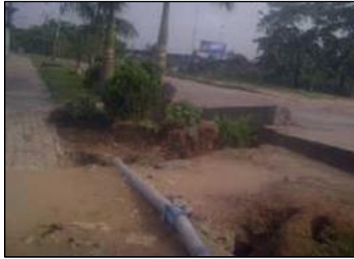
Figure 1 Poor drainage resulting in the separation and disjoint of access route
