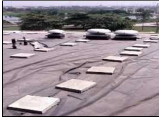
Figure 3 Covering of roof felts with damp proof membrane due to high rate of leakages
