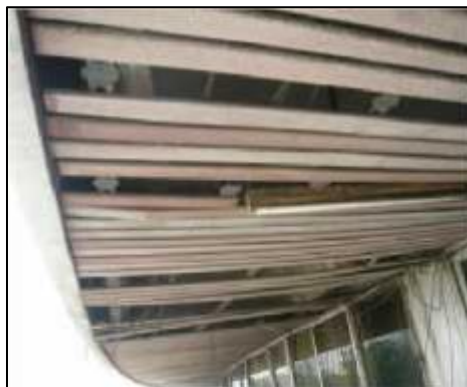
Figure 6 Damaged suspended ceiling rails with visible rust
